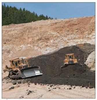
Stockpiled topsoil can be performance-boosted with pumice to enhance drainage and mitigate runoff while supporting vigorous plant cover.
