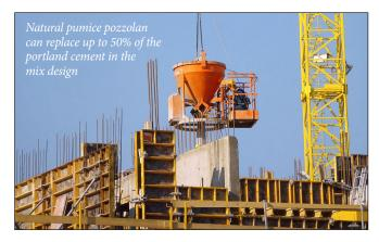
R-value for the same width of standard-aggregate concrete wall is increased 4 times, and the thermal mass benefits still remain. With the increased R-value inherent in the pumice concrete walls themselves, additional insulation needs go down.
